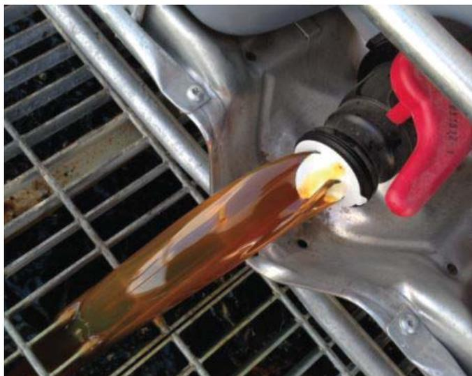
ENERLUBE was added directly to the suction pit, adjusting the tote valve to control the rate of addition
