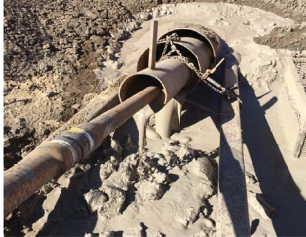
ESL HDD is used to elevate viscosity in the EnerSEAL HDD system
