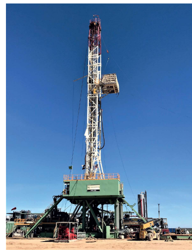
Drilling rig, located in Reeves county
