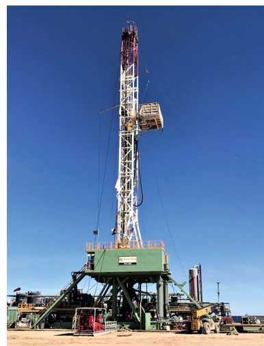
Drilling rig, located in Reeves county
