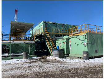
Figure 1: Stacked generators and pump houses reduce footprint
