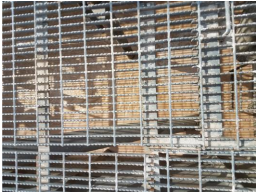
Image 5: Yard mix tank from the top grating
