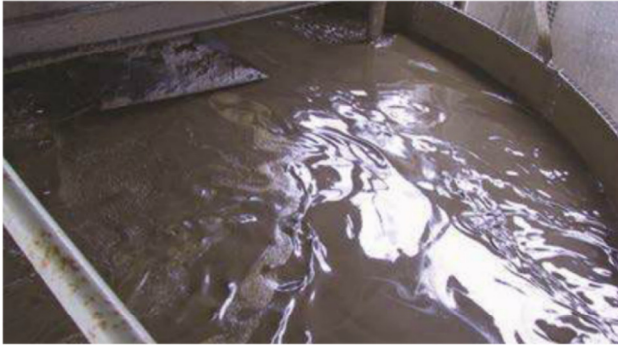
Figure 2. Invert oil base mixing plant in Benwood, West Virginia.
