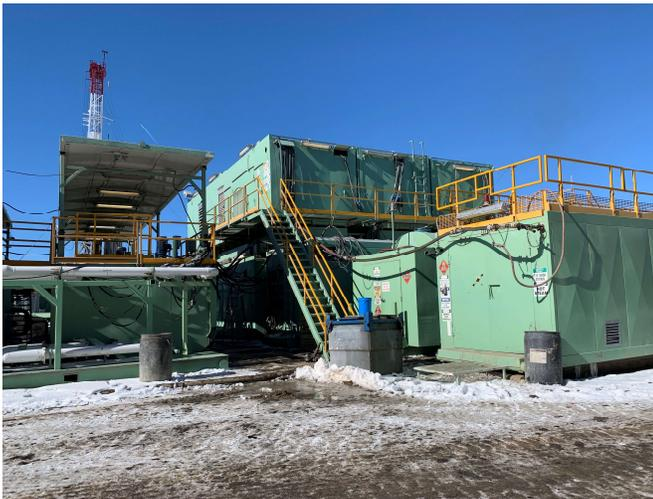
Figure 1: Stacked generators and pump houses reduce footprint
